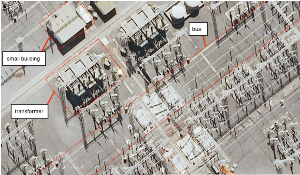
Figure 9: Otahuhu substation showing transformer T12, with a small building indicated for size comparison (this picture is from Google Maps).
